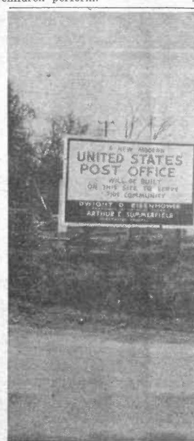
NEW IUKA POSTOFFICE CONSTRUCTION — Slow progress is being made on construction of the new U. S. Postoffice building in Iuka. Delay has been caused in part by difficulty in obtaining materials and partly because of adverse weather conditions. The original target date for completion of the building was November 15. It will now probably be February 1961 before the building is finished, a spokesman stated.
